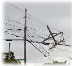
Figure 8: Seabrook Pole Damage
