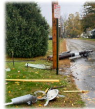
Figure 7: Concord Pole Damage
